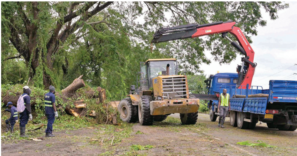
Workmen from the National Solid Waste Management Authority (NSWMA) use heavy equipment to clear a section of the Mandela Highway at the Portmore intersection on Wednesday (Oct. 29). Fallen trees and other debris from the passage of Hurricane Melissa, had left the westbound section of the Highway, towards Spanish Town, impassable.
