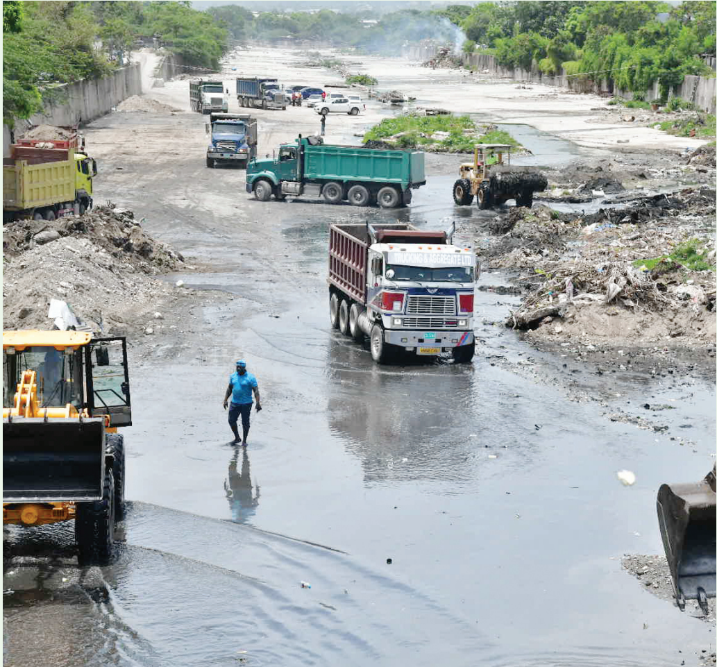
The National Works Agency (NWA) team using heavy equipment to clear the Sandy Gully in the vicinity of Spanish Town Road in Kingston. The Government has allocated $2 billion to undertake comprehensive gully works.
