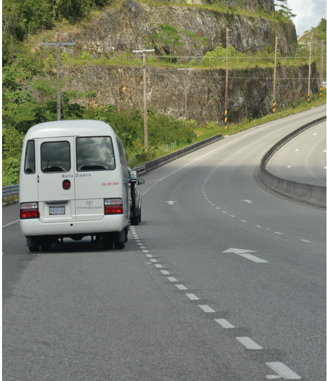
A section of the North-South Highway, which spans St. Catherine and St. Ann
