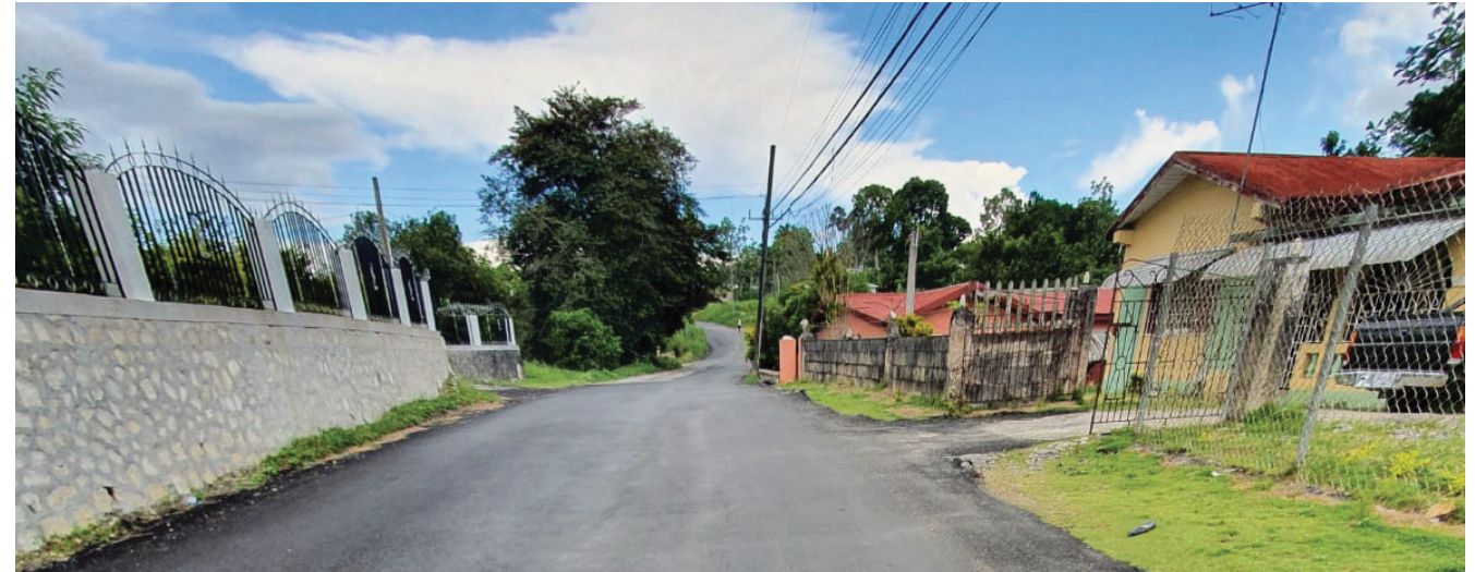
A section of the newly-rehabilitated Whithorn to Darliston roadway in Westmoreland.
