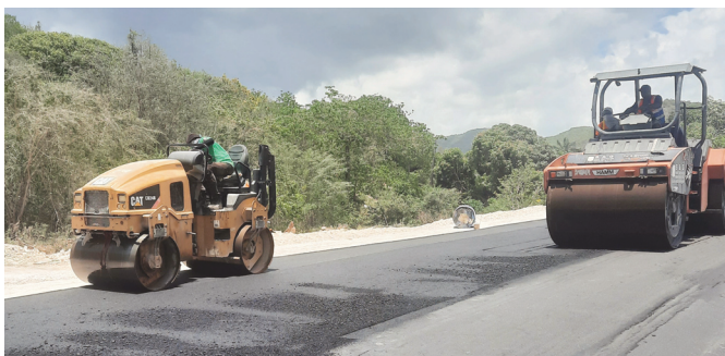
Paving works on a roadway in rural Jamaica.
