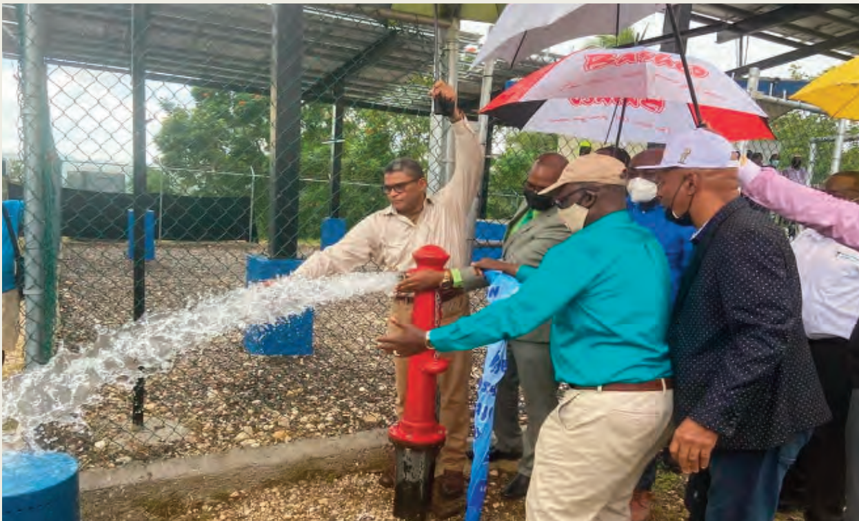
Commissioning of the Top Aberdeen Water Supply System in St. Elizabeth.
