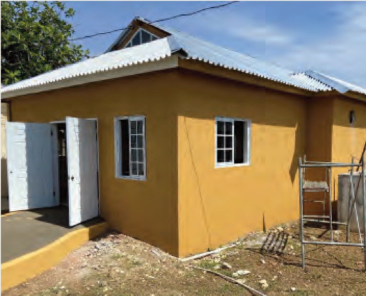
Newly constructed kitchen at the Hanover Infirmary.
