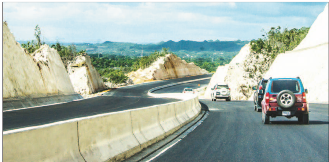
A section of the newly constructed North-South Highway
